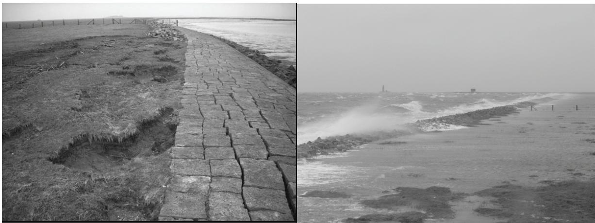
Figure 1: Scouring at the existing revetment (left), overtopping during storm tide (right) (Photos: N. Kumbruck).
